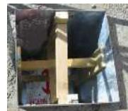
Shore the inside of the casing before pouring the concrete to avoid any deformation of the casing.
